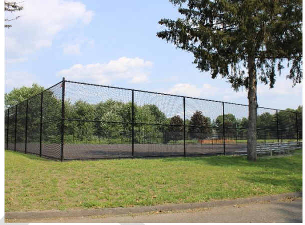
Figure 13: Tennis courts at Blunt Park, subject of an ongoing rehabilitation project.
